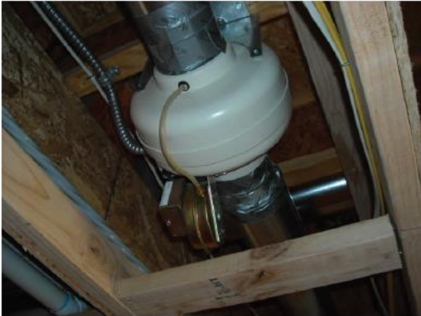
Dryer exhaust duct power ventilator (DEDPV)
